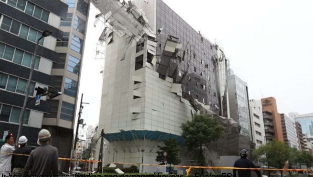
It brought down scaffolding and damaged houses -- Photo: EPA
